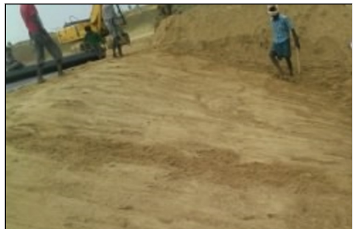
Photo 1: Dressing of slopes of the pond
