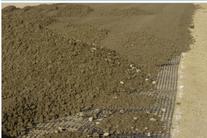
Photo 3: Laying of GSB over ParaLink®
