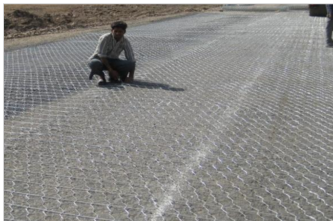
Photo 6: Laying of Road Mesh®
