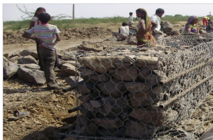
Photo 2: Gabion wall embankment edges
