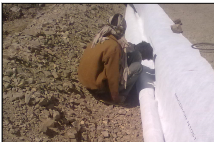
Photo 5: Installation of MacDrain® for drainage
