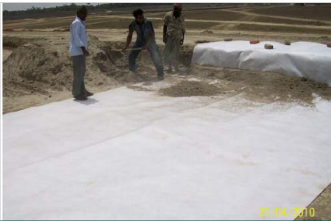
Photo 3. Sand filling on Geotextile
