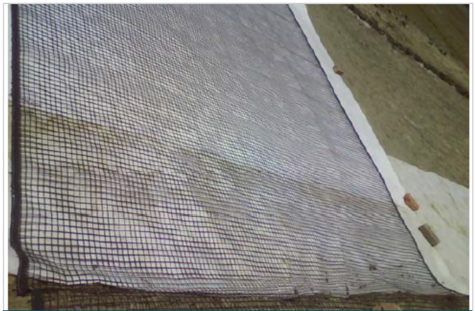
Photo 4. Laying of MacGrid WG4S
