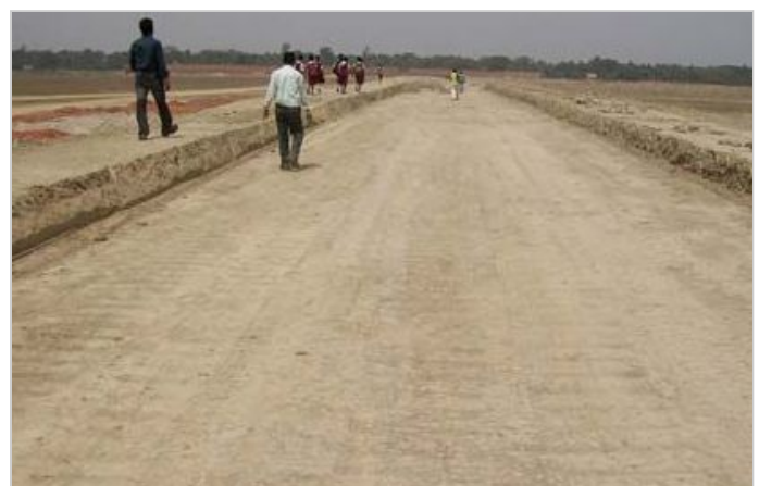
Photo 2. Embankment ready for laying MacTex H
