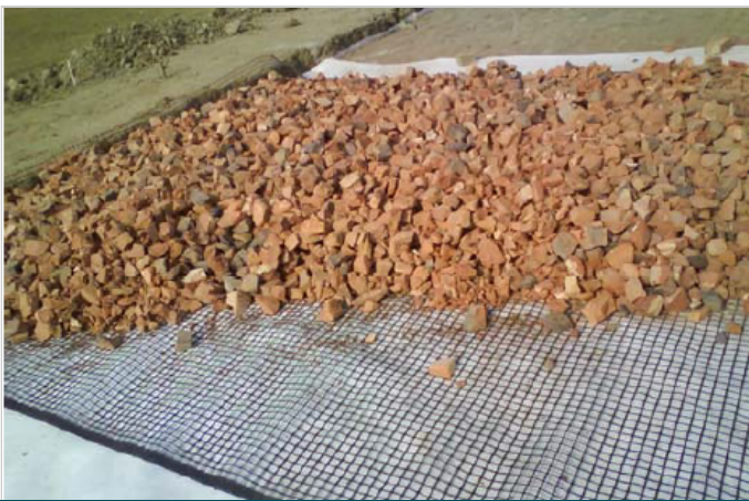
Photo 5. Laying of Jama Khoa over MacGrid WG4S
