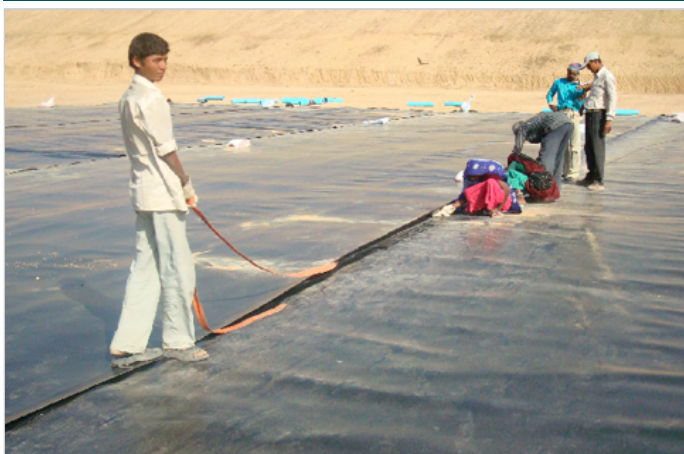
Photo 3. Joining of adjacent membranes by wedge welding
