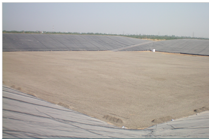
Photo 6. Base liner and side liner laying completed
