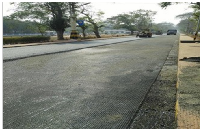
Photo 2: MacGrid® AR installation
