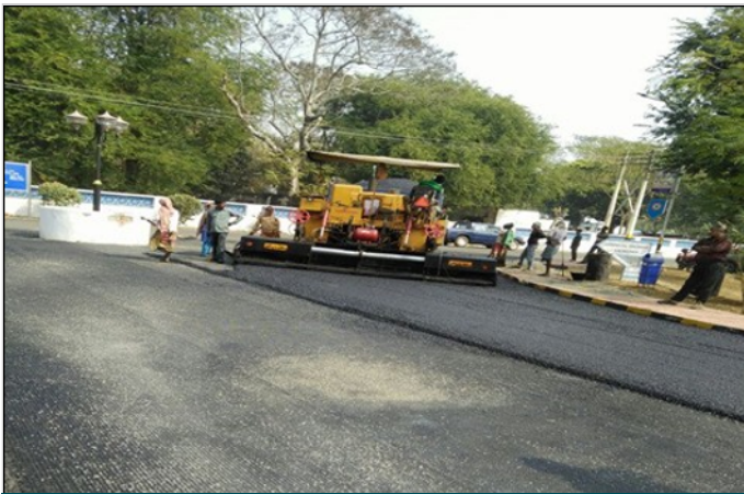
Photo 5: Construction of overlay
