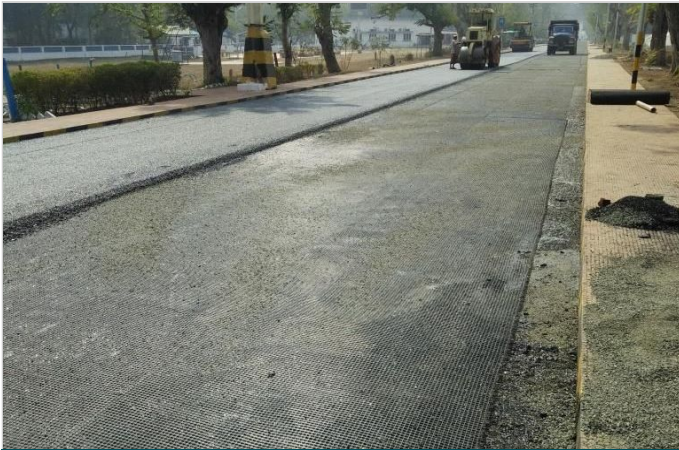
Photo 3: MacGrid® AR installation completed
