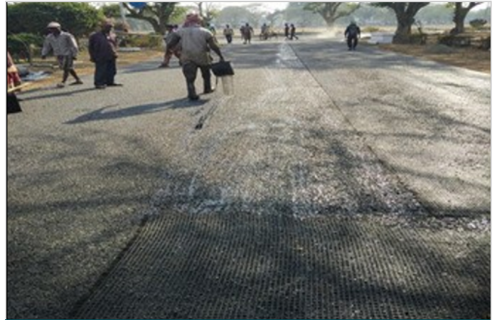
Photo 4: Photograph showing the tack coat application prior to overlay
