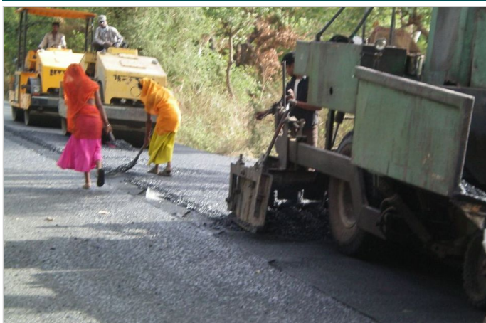
Photo 3: Laying of 20mm thick SDBC layer
