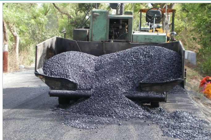
Photo 5: Laying of 75mm thick BM layer
