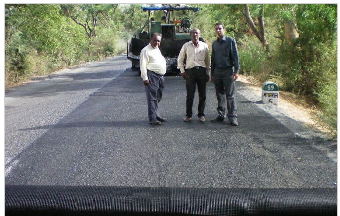
Photo 2: Laying of MacGrid® over BUSG layer
