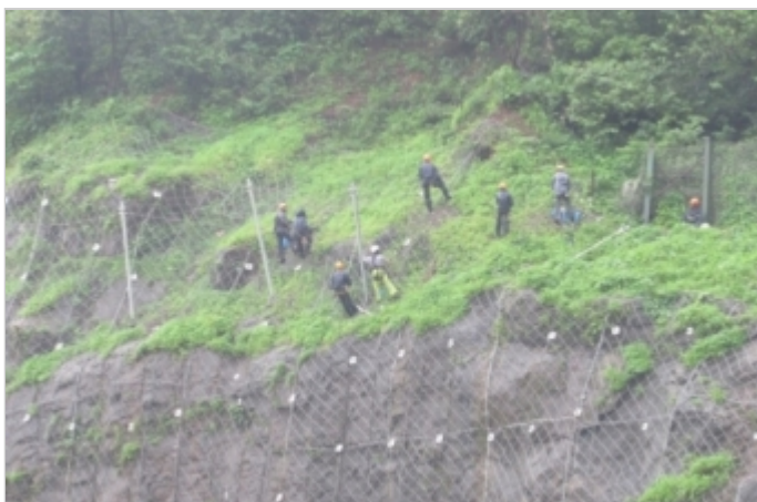
Photo 5: Rockfall mitigation measures at Adoshi tunnel- Dynamic Rockfall Barrier
