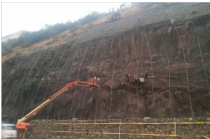
Photo 3: Rockfall mitigation and slope stabilisation measures
