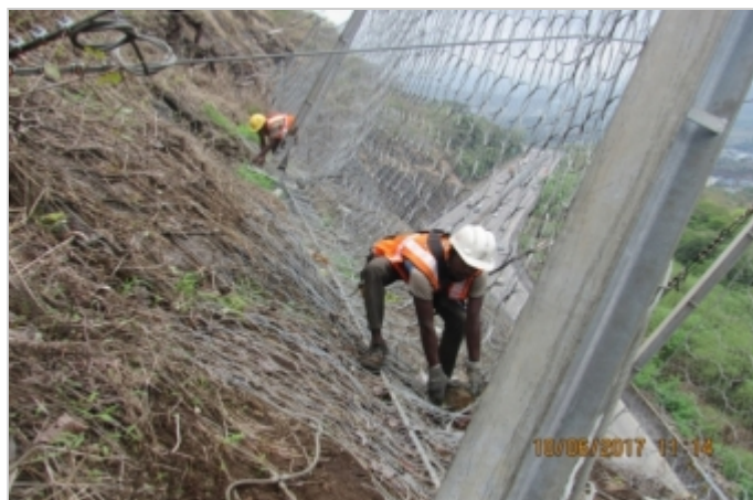
Photo 6: Cleaning off the debris from upslope side of the rockfall barrier
