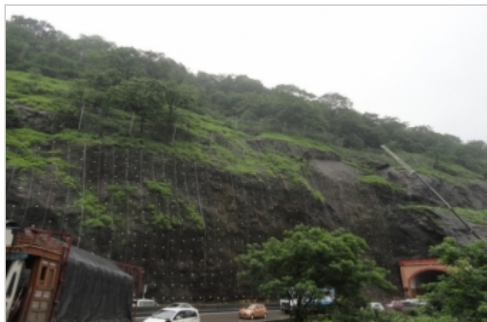
Photo 4: Rockfall mitigation measures near Adoshi tunnel
