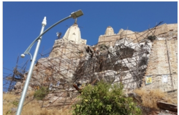
Photo 1: Scaffolding at site for anchoring.
