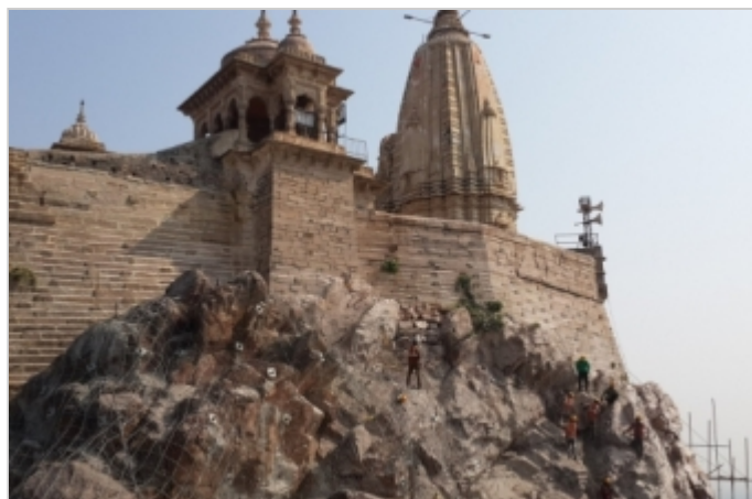
Photo 6: Mesh installation at the back side of temple
