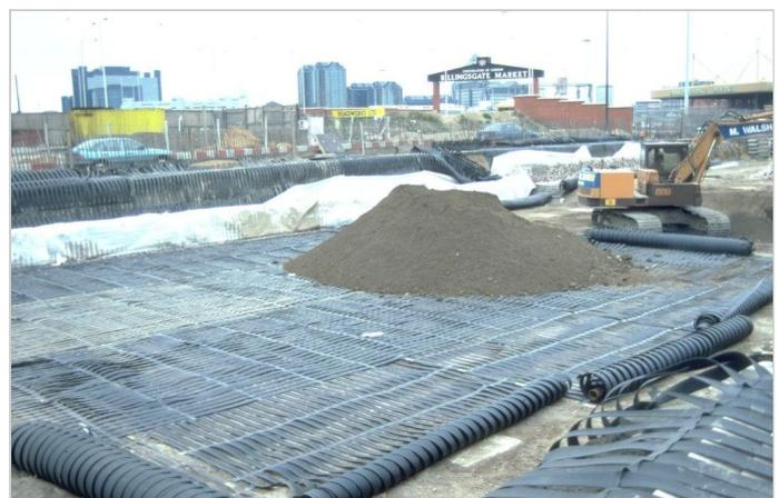
PFA was used as fill to create the embankment
