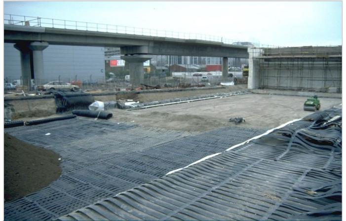
Backfilling in operation over the Paralink LTP
