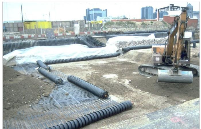
Paralink placed in two direction over the pile caps
