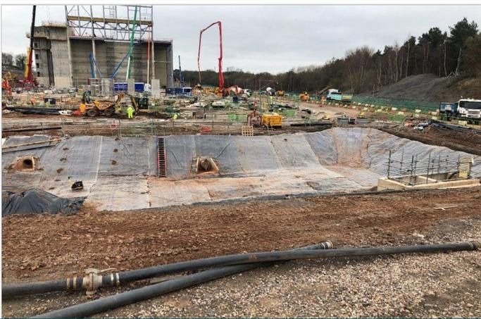
Macline GCL W20 being installed within the attenuation pond located to the rear
