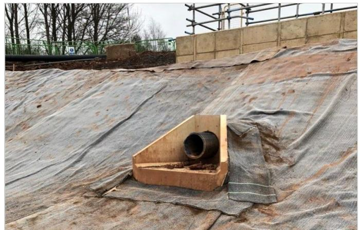
Macline GCL W20 patch panels placed to seal the interface around the headwall.
