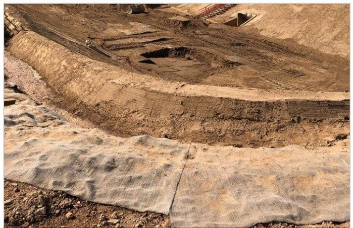
Macline GCL W20 is anchored at the crest of slopes in a trench.
