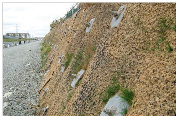
MacMat® R and soil nails after hydroseeding
