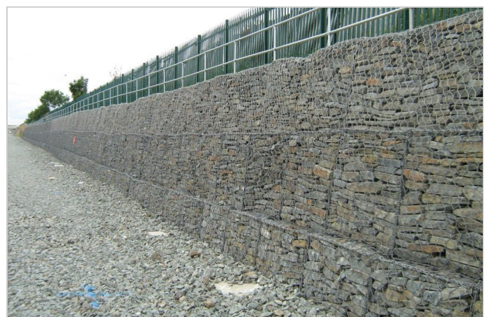
Installation of Gabion retaining wall
