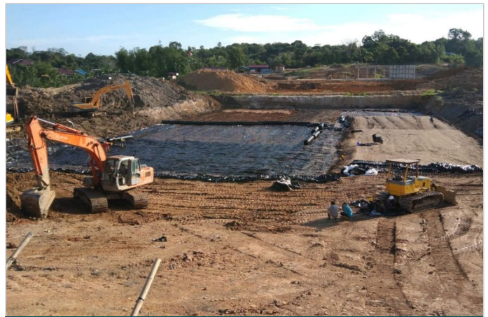
Geogrid Laying in Biaxial Direction
