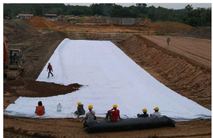
Geotextile Laying
