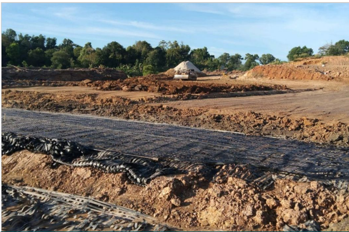
Geogrid Laying in Biaxial Direction
