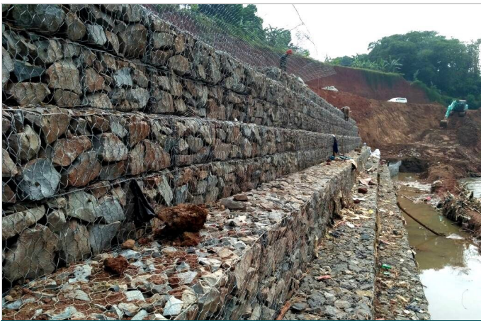
Installation of Terramesh®
