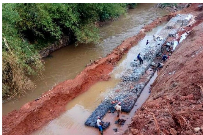
Installation of Reno Mattress® as scour protection
