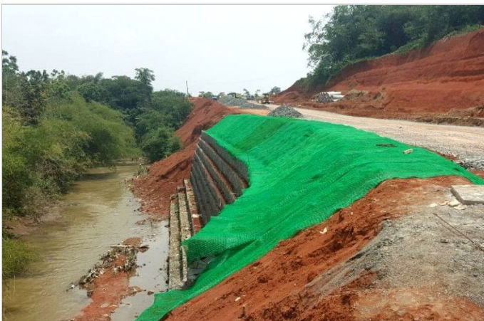
Installation of MacMat® as erosion control
