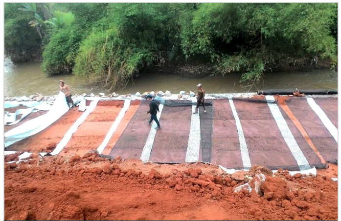
Installation of MacGrid®
