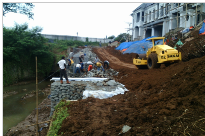
Gabion retaining wall during construction
