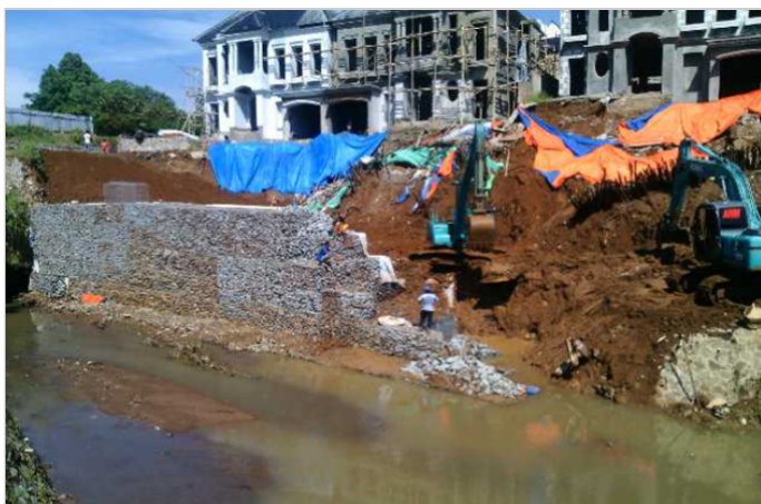
Gabions and Reno Mattresses during construction
