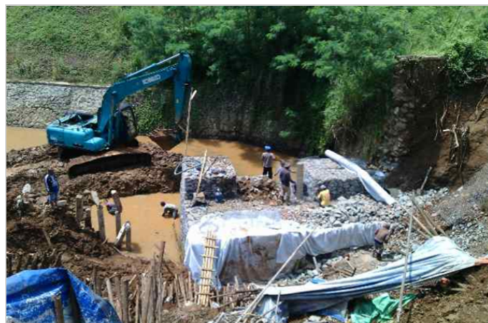
Gabion retaining wall during construction
