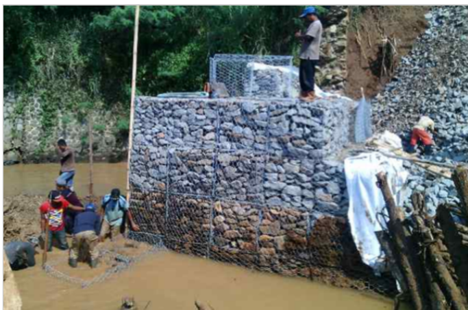
Reno Mattresses installation as scour protection
