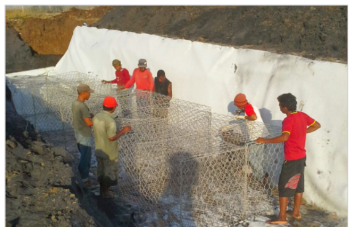
Gabion Installation
