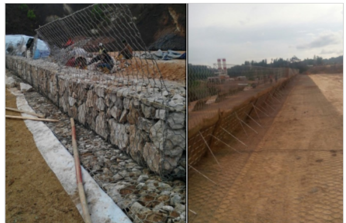
Terramesh & Green Terramesh Installation
