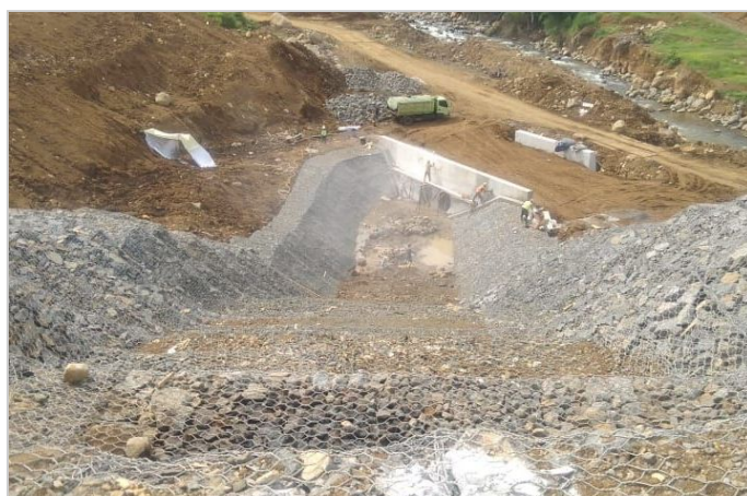
Installation process of Gabion and Reno Mattress
