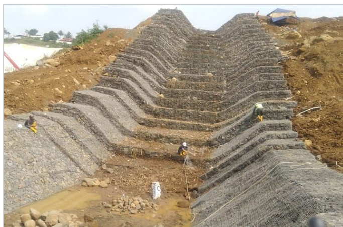
Installation process of Gabion and Reno Mattress
