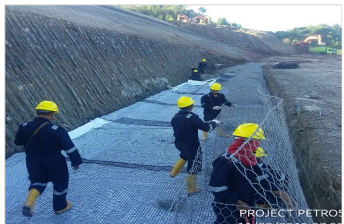
Terramesh System Installation
