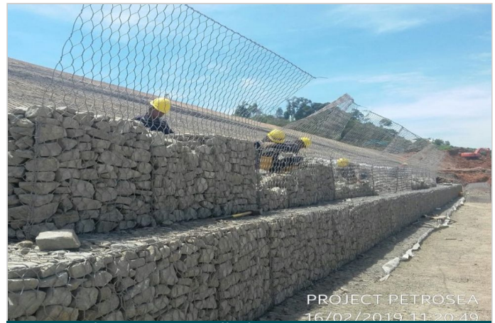
Terramesh System Installation
