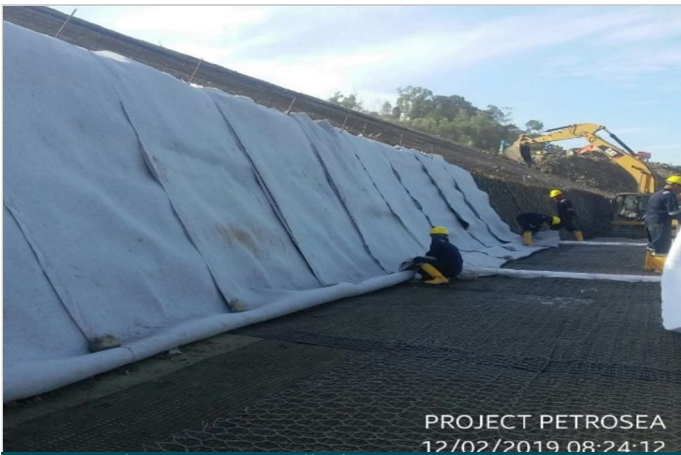
Terramesh System Installation
