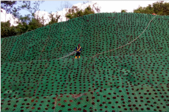
Application of Mulching on Macmat HS
