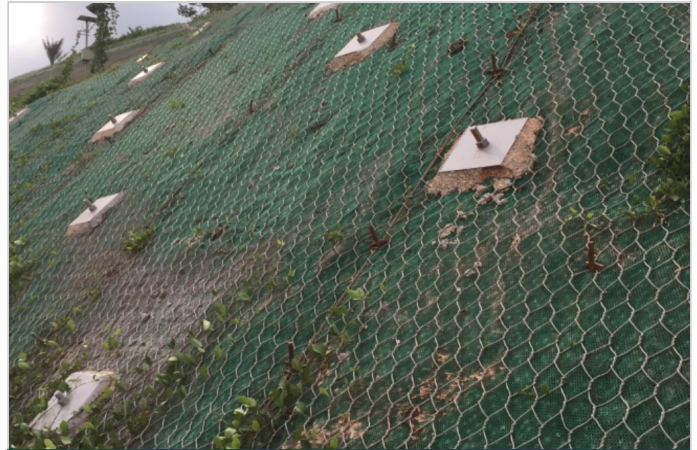
Soil Nailing application on Macmat HS
