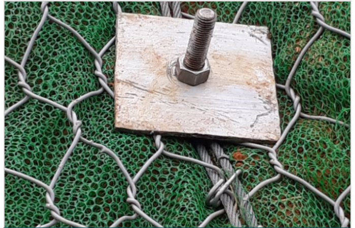
Soil Nailing application on Macmat HS
