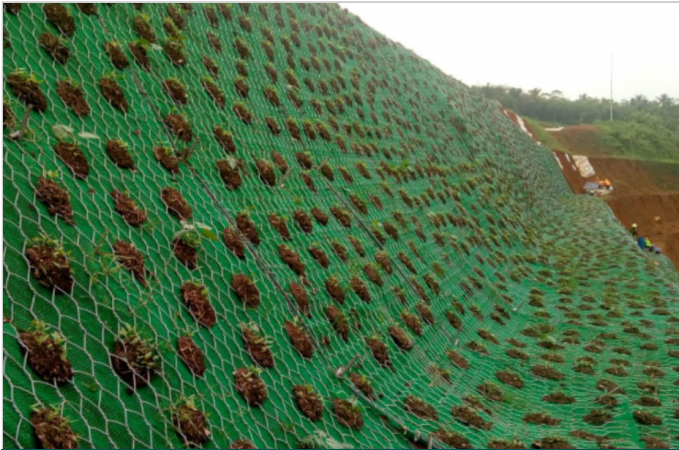
Application of Mulching on Macmat HS
