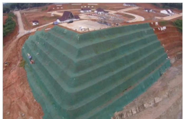
Overview of Installed Macmat HS
