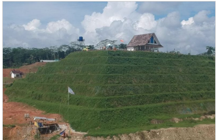
Condition of Installed Macmat HS in March 2019
