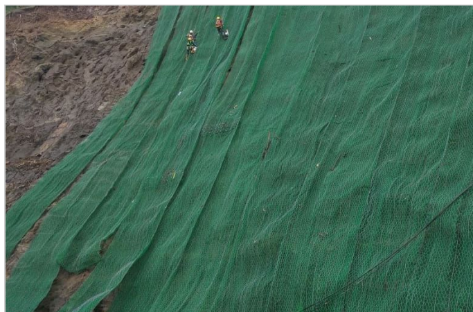
Installation process of Steelgrid® HR 30 + MacMat® EM as netting
