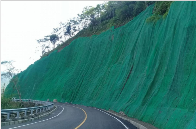
General view of installed drapery system
