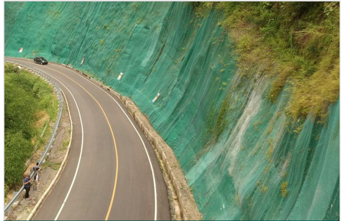
General view of installed drapery system
