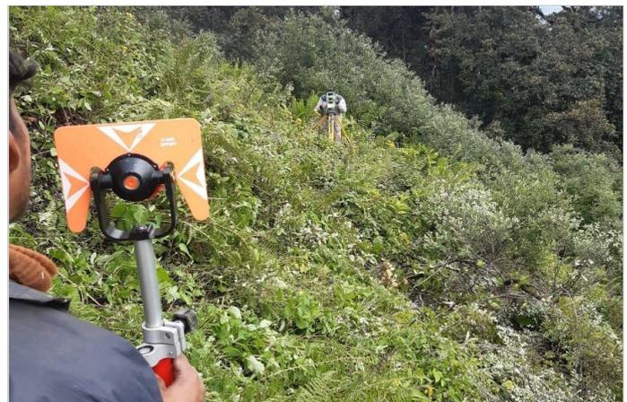
Figure 1-Survey ongoing for alignment fixing
