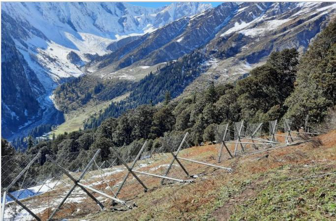
Figure 5-Multiple lines of Snow ErdoX lines installed (view from upslope)
