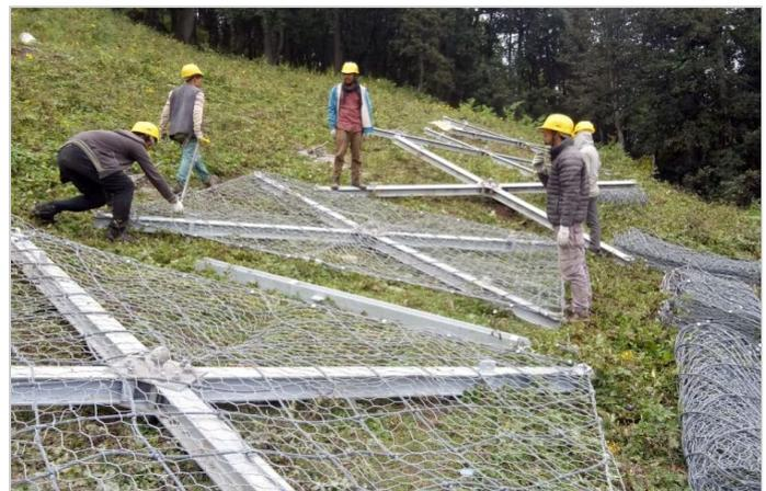
Figure 2- Onsite fabrication of individual Snow ErdoX unit
