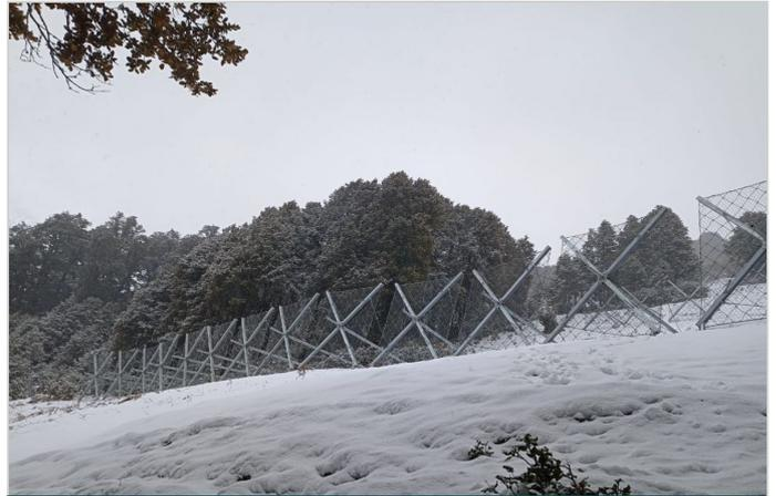
Figure 4-Multiple lines of Snow ErdoX lines installed (view from downslope during)
