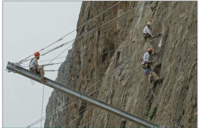
Figure 4- Installation of dynamic rockfall barrier
