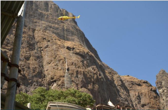
Figure 3- Helicopter used to transfer material during installation
