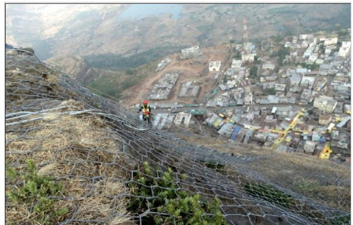
Figure 1- Steelgrid MO laid out on slope surface
