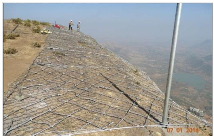
Figure 2-HEA Panels laid over Steelgrid MO on slope surface
