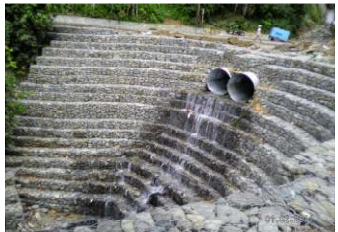
End of construction
