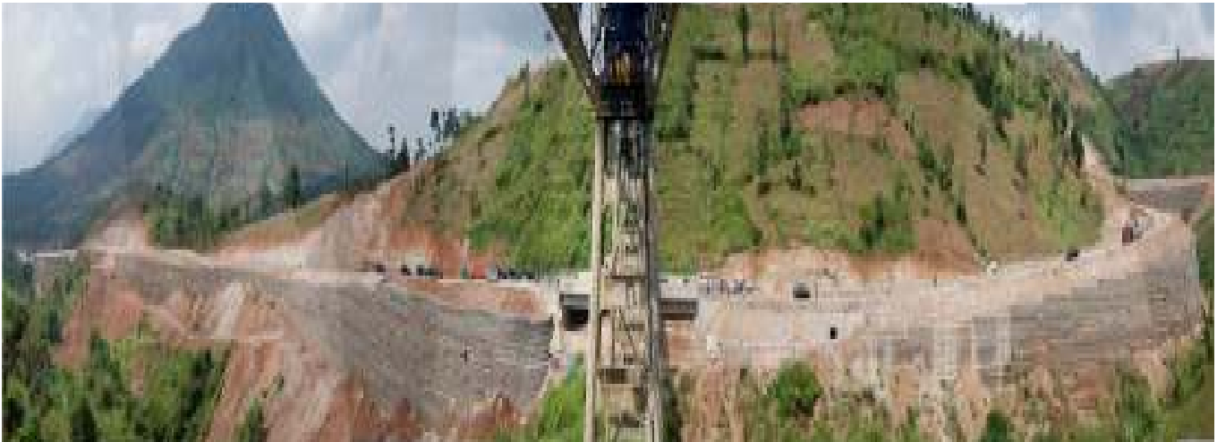
End of Construction
