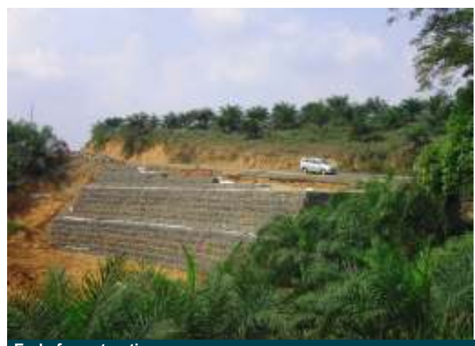
End of construction
