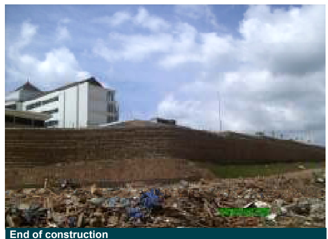
End of construction
