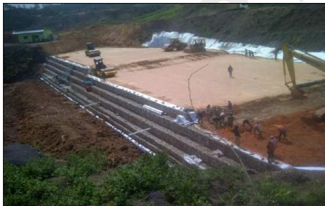
Stage 1, progress in December 2015
