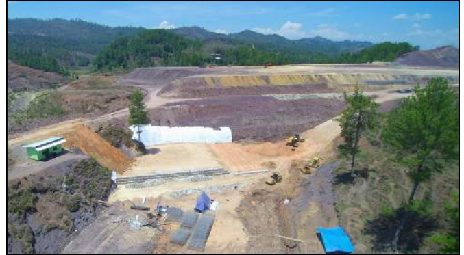
Aerial photo of the Paramesh under construction, Nov 2015
