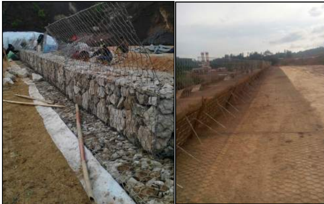
Terramesh System and Green Terramesh installation
