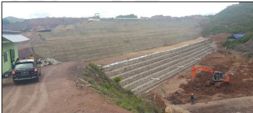
Stage 1, progress in January 2016
