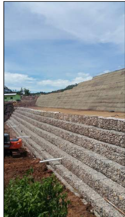
Stage 1 completed, February 2016
