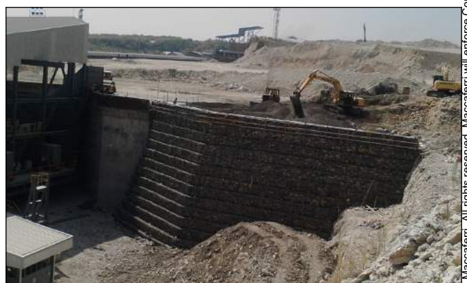
Wall after completion
