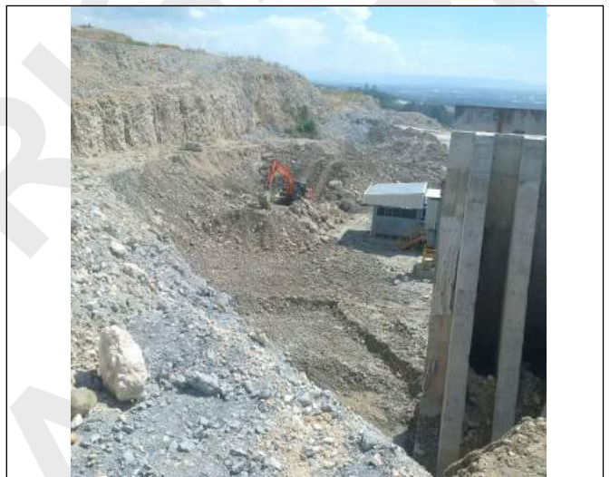
Site condition before the construction
