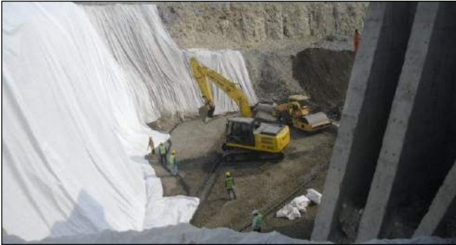
Installation of the filtering geotextile for the drainage system
