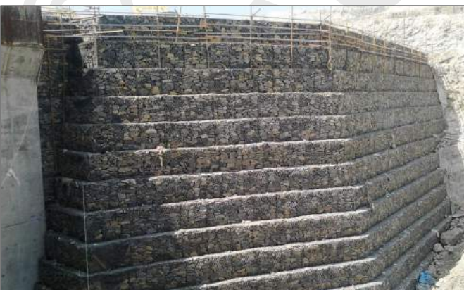
Wall after completion
