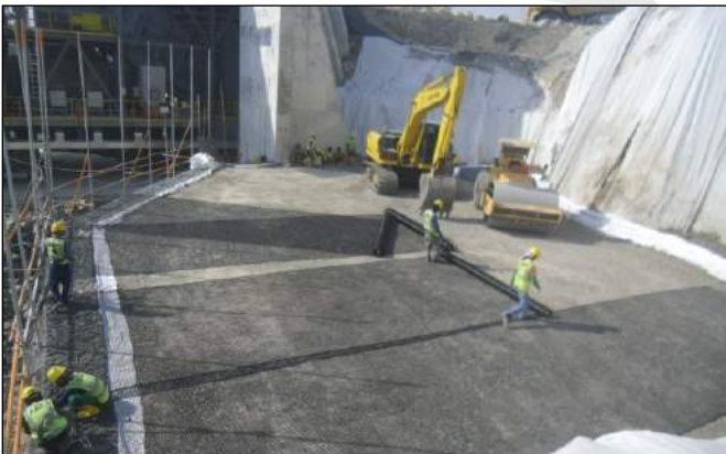
Laying MacGrid WG 15
