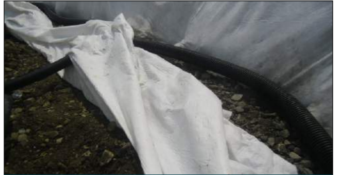
Stones as draining material; Corrugated collecting pipes
