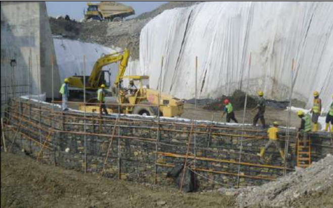
Terramesh System installation
