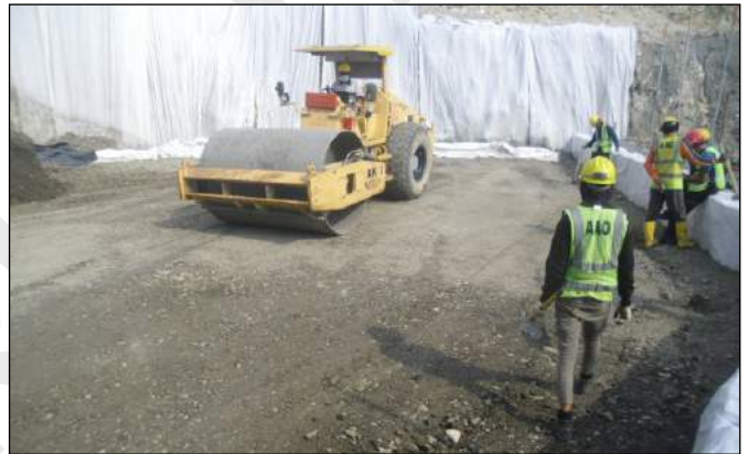
Compacting operations
