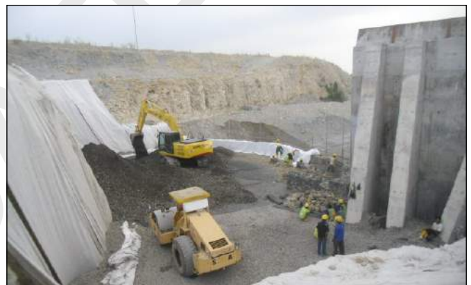
Backfilling with granular material
