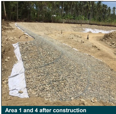
Area 1 and 4 after construction
