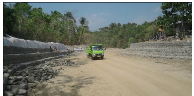
Area 2 and 3 after construction
