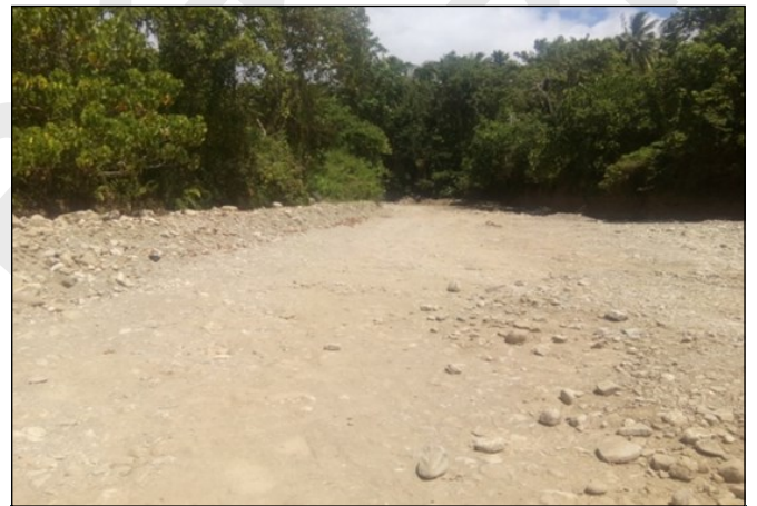
River condition before the intervention
