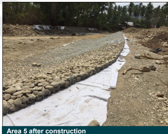
Area 5 after construction
