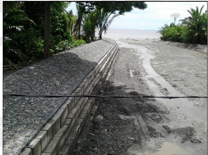
Area 1 and 4 after construction
