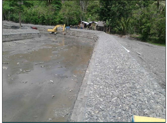
Area 1 and 4 after construction
