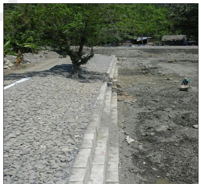
Area 2 and 3 after construction
