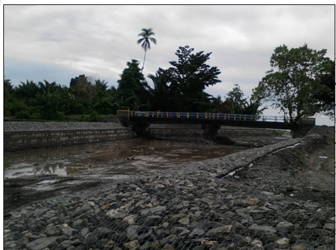
Area 1 and 4 after construction
