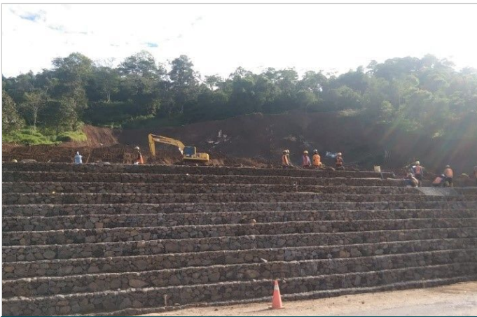
Installation of Terramesh
