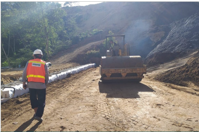
Embankment Compaction
