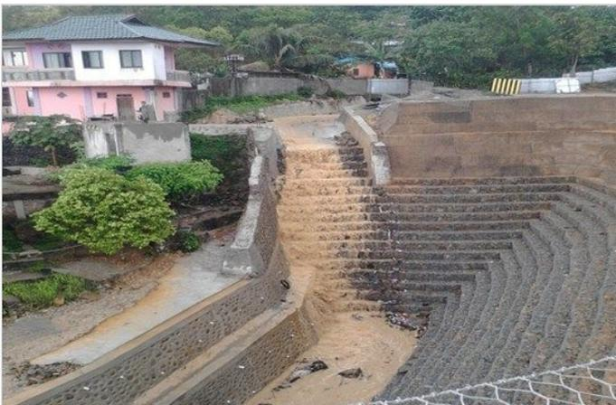
Drop structure working during a flood event
