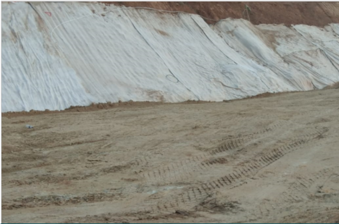
Installed Macline GCL W10 on the existing slope
