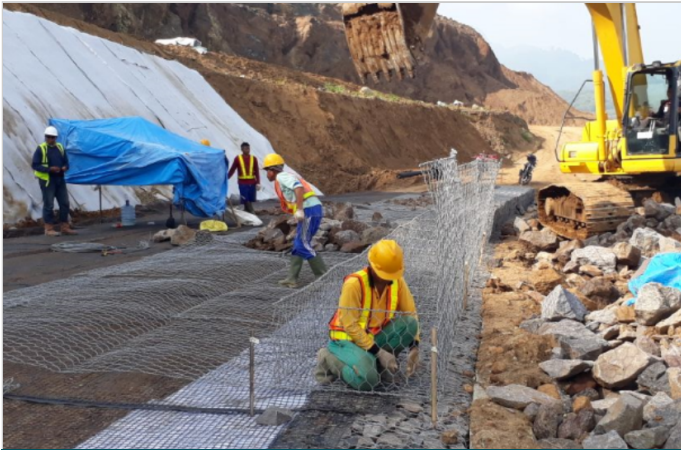
Installation of Terramesh System and MacGrid WG
