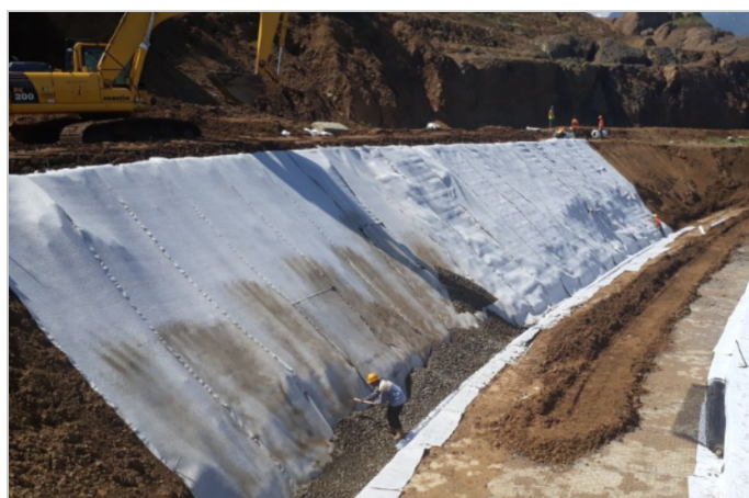
Installation of MacDrain as subdrain
