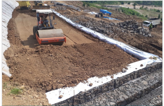
Compaction process of the structural fill
