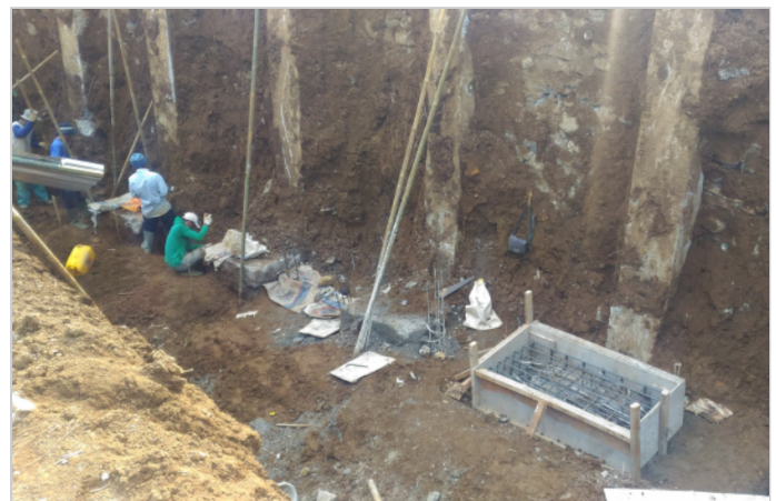
Bored piles construction under the masonry wall
