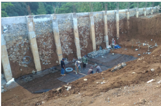
Installation of first layer of Terramesh and MacGrid WG
