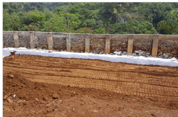
MacTex MXS 250 as Separator between Backfill and Terramesh
