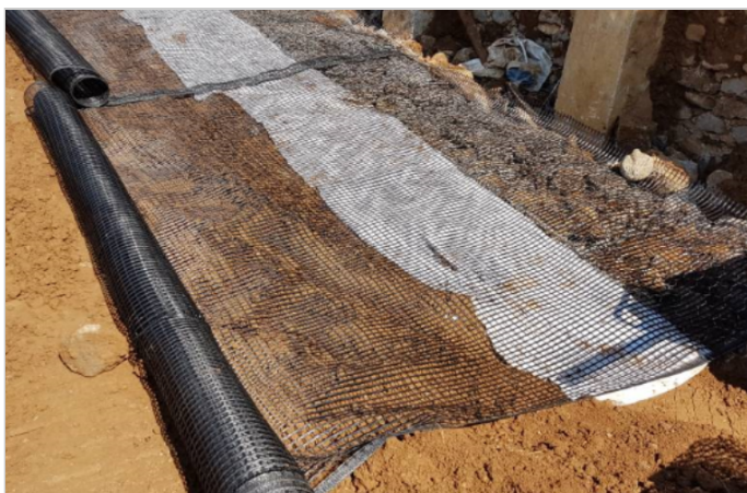
Installation of MacGrid WG20
