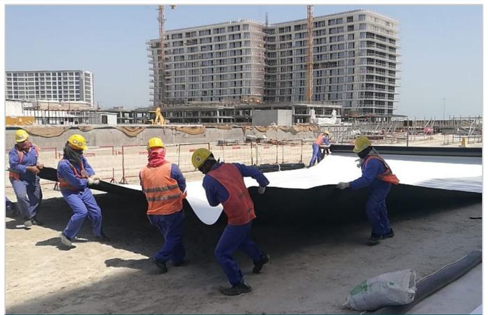
During construction: deployment of Macline geomembrane layer
