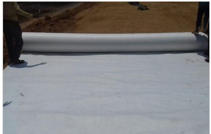
Photo 1: Laying of MacTex N at blanket & subgrade interface
