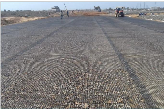
Photo 3: Laying of MacGrid EG at middle of blanket layer
