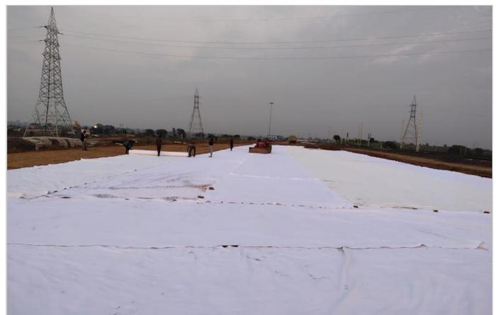
Photo 2: Laying of MacTex N at blanket & subgrade interface
