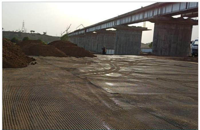
Photo 4: Laying of MacGrid EG at middle of blanket layer
