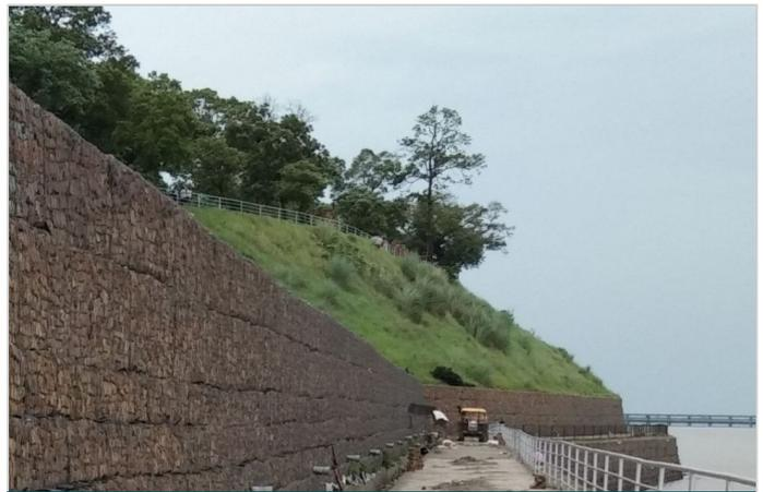
Figure 4-Vegetated surcharge slope covered with MacMat R (Paramesh wall)
