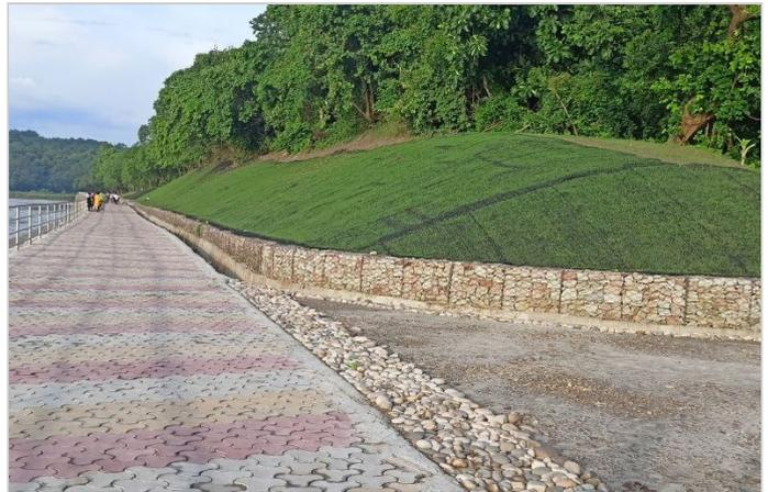
Figure 6-Vegetation establishment over MacMat R installed slope
