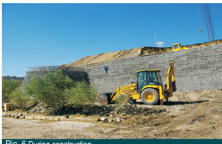
Pic. 6 During construction
