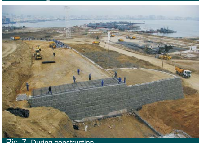
Pic. 7 During construction
