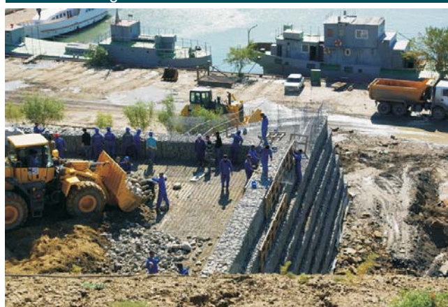
Pic. 5 During construction
