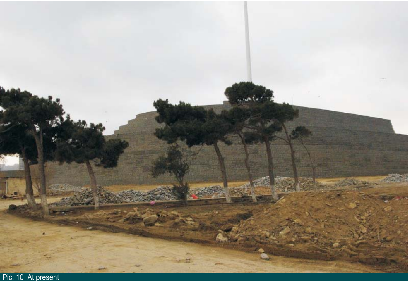
Pic. 10 At present
