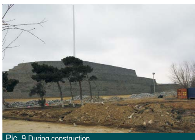
Pic. 9 During construction
