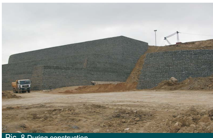
Pic. 8 During construction
