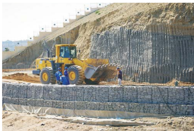
Pic. 4 During construction
