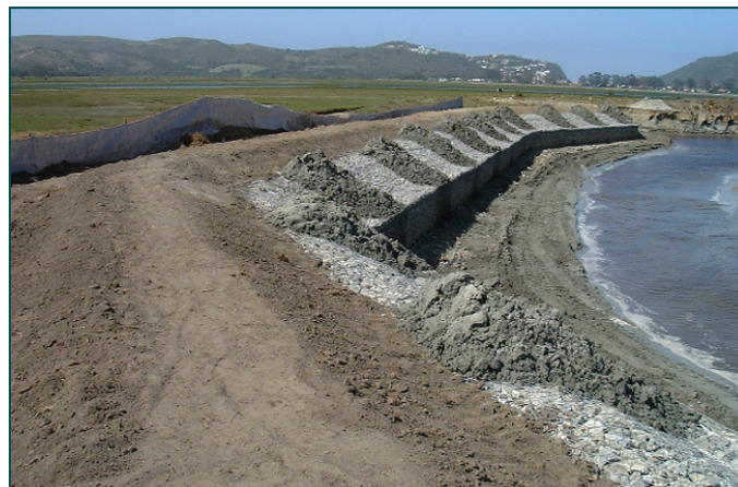
Toppingsoiling of Reno mattresses
