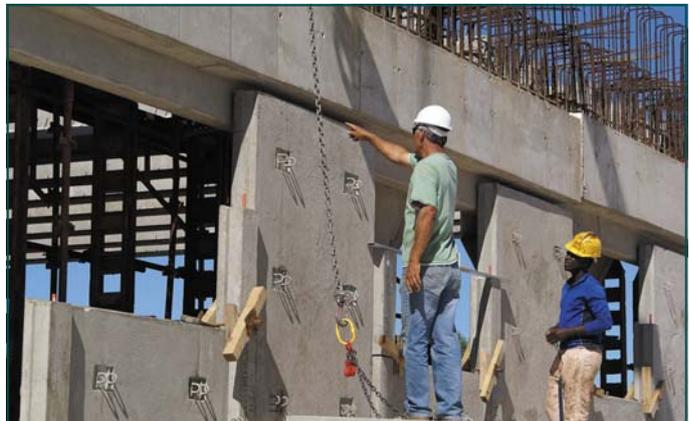
Checking clearance between MacForce panel and bridge
