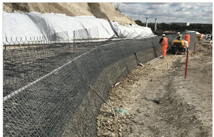
Mineral Terramesh units being erected - Note MacDrain to rear
