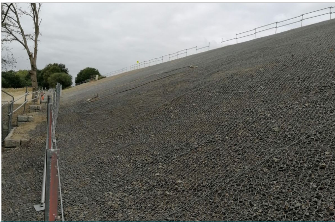
Area covered with the protective mesh
