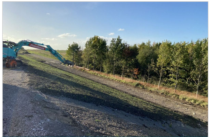
Topsoil laid on top of the mesh foundation
