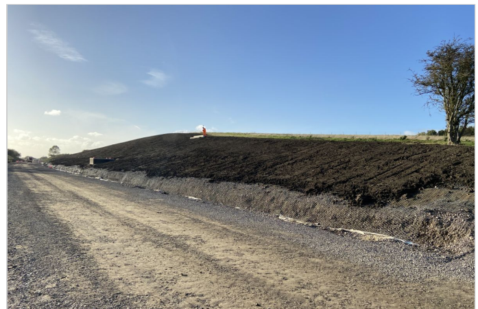
Anti-burrowing DT Mesh spread across rail embankment
