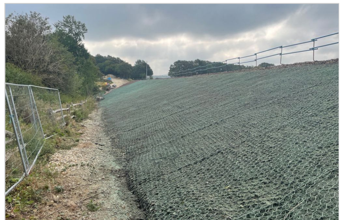
Anti-burrowing DT Mesh deployed and secured
