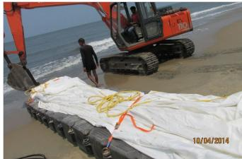
Photo 4: Transfer of tubes into the sea using pontoons
