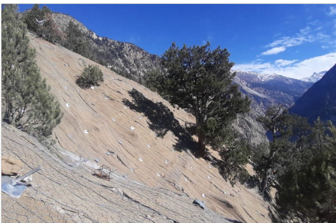
Figure-5-Installed Steelgrid and jute mat
