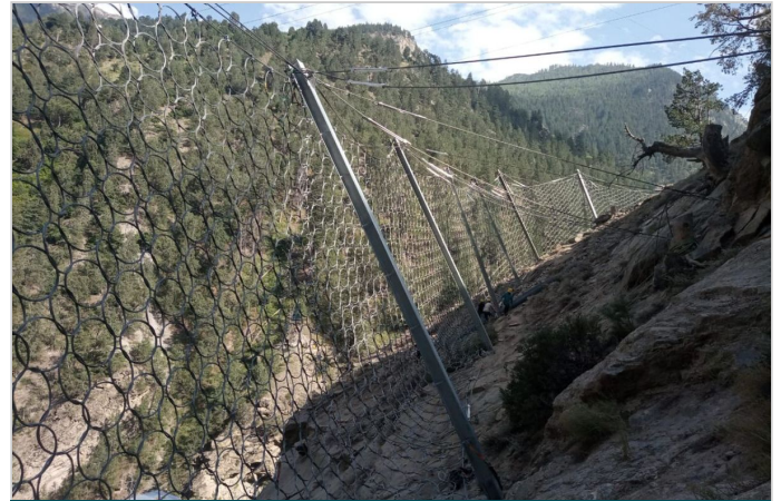
Figure-4-Installed dynamic rockfall barrier.
