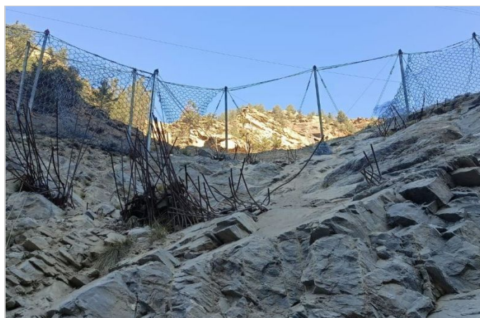
Figure-2-Dynamic rockfall barrier during construction
