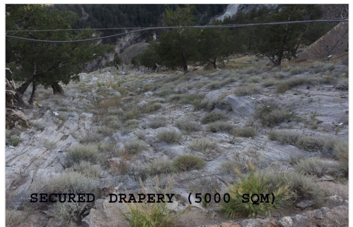
Figure-6-Installed Steelgrid and jute mat
