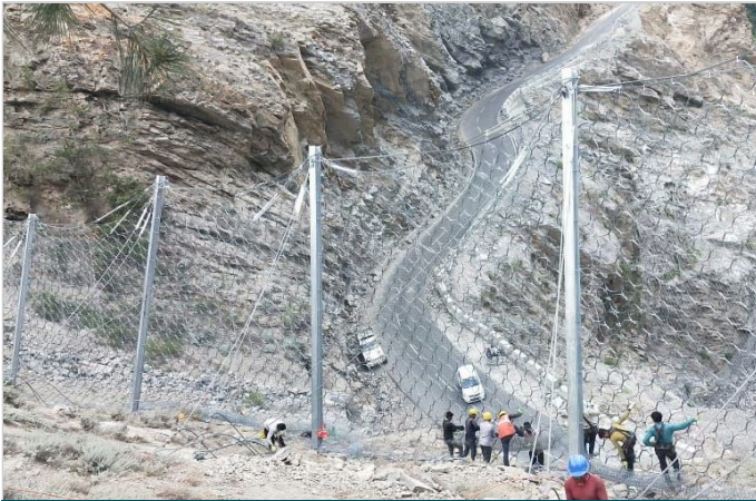
Figure-3-Installed dynamic rockfall barrier
