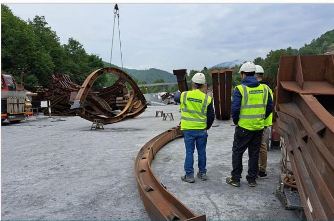
Pre-assembled Automated Tunnel Rib HEB300
