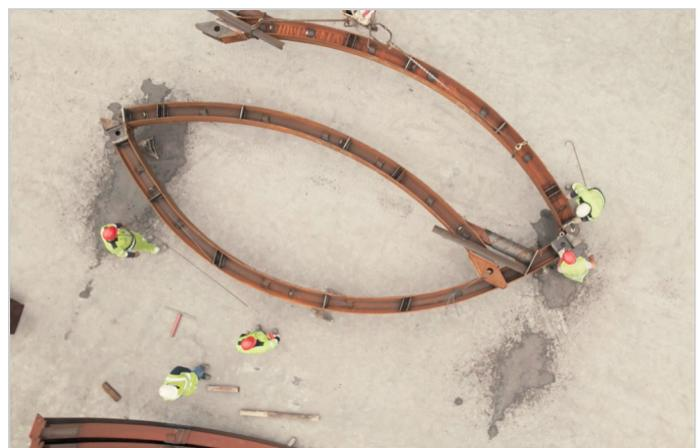
Crown and shoulder sections are pre-assembled with the hinge
