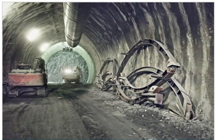
Pre-assembled Automated Tunnel Rib HEB300 before installation
