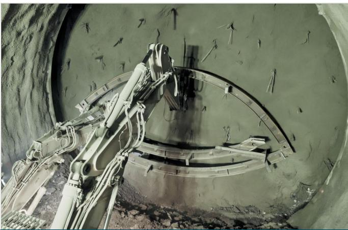
Automated installation with no workers near the excavation face
