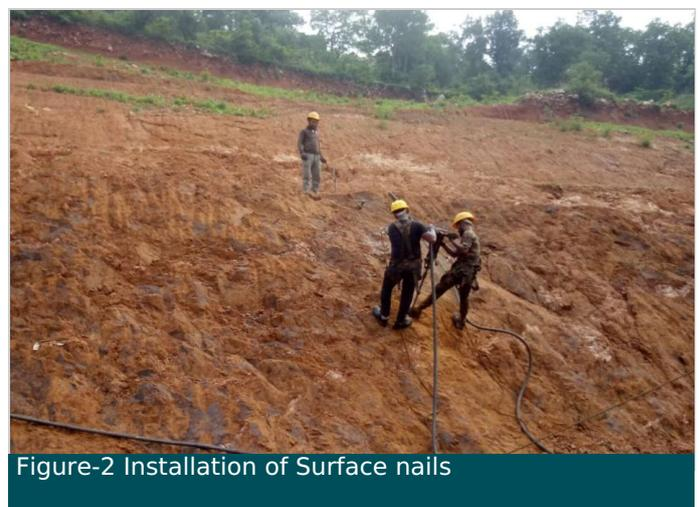
Figure-2 Installation of Surface nails
