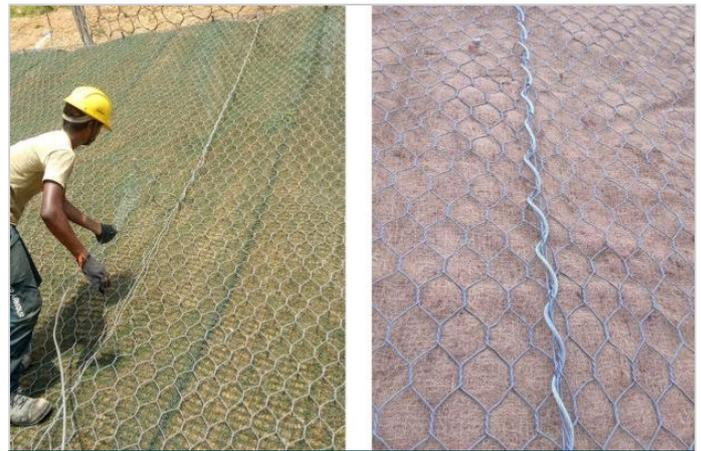
Figure-4 Installation of wire rope vertically on the edges of DT mesh
