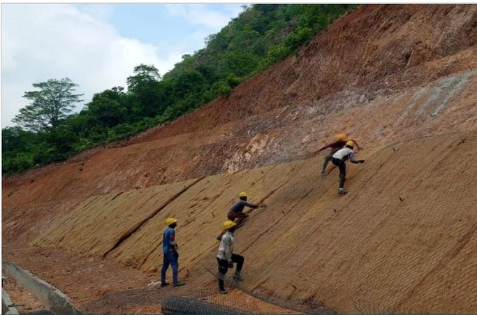
Figure-3 Providing DT mesh over the erosion control mats
