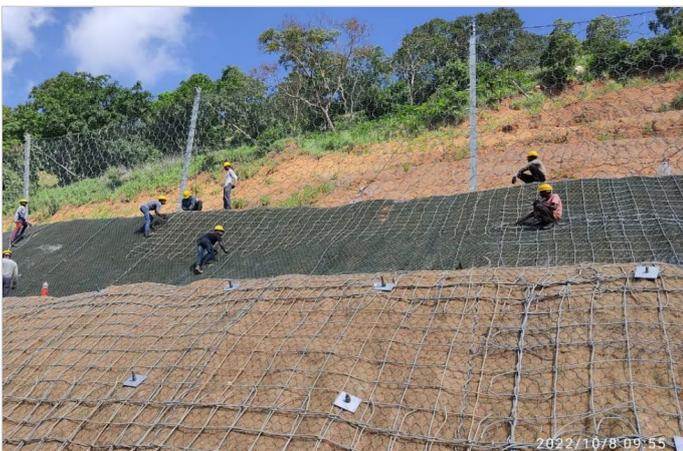
Figure-5 Mesh installation over nailed slope face
