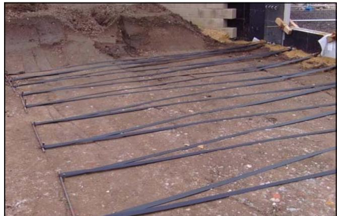
Typical deployment of Paraweb strip reinforcement
